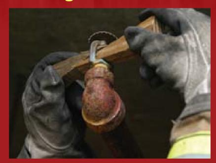
Step 2: Insert the two wedges, one from each side, between the discharge orifice and the sprinkler head deflector.
