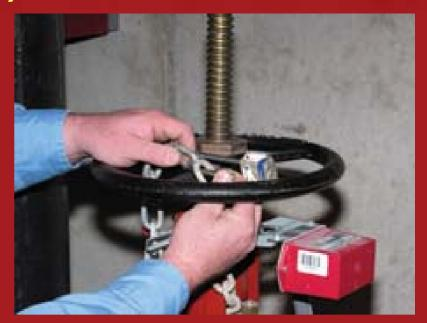
Step 3: To open the OS&Y valve, turn the handle counterclockwise until resistance is strong and the stem is visible again. Lock the valve in the open position.
