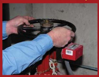
Step 2: Turn the valve handle clockwise to close the valve. Keep turning until resistance is strong and little of the stem is visible.
