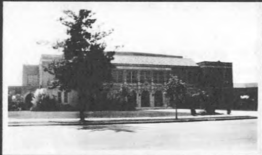
Glendale Union High School First home of Glendale College
