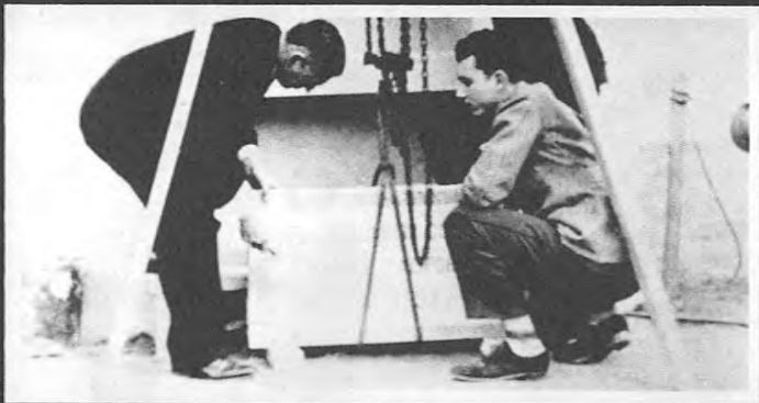
Judge W. Jurney and Ted Robinson laying corner stone — Dedication, 1937
