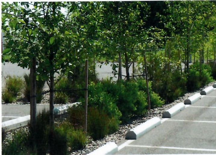
Parking lot - Stormwater man-
