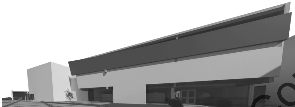
View of the Exterior Front (Mall)
