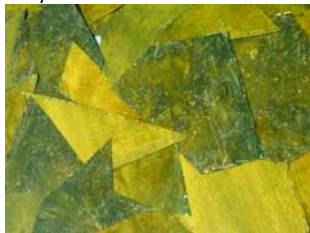
The detail of the copper skin
